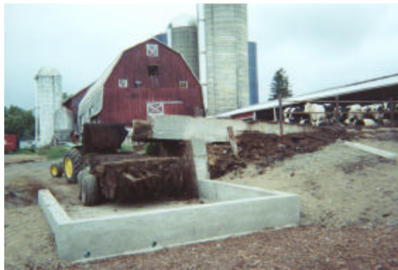
Figures 10 and 11. Leubner Farm Post-BMP Manure Handling Station
